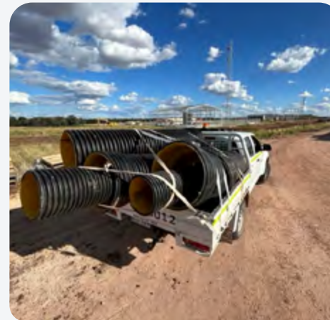
Blaxmax pipes were collected to be used as small road crossovers.
