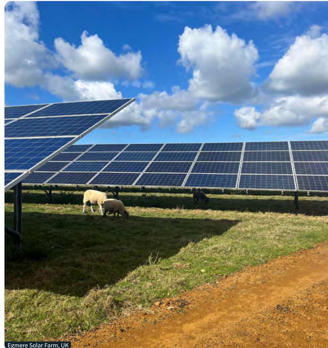
Egmere Solar Farm, UK
